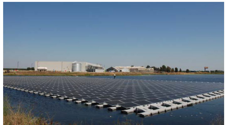
Figure 7. Aerial view of Salad Cosmo's pond and floating solar plant. Source: Google maps and Ciel & Terre.
